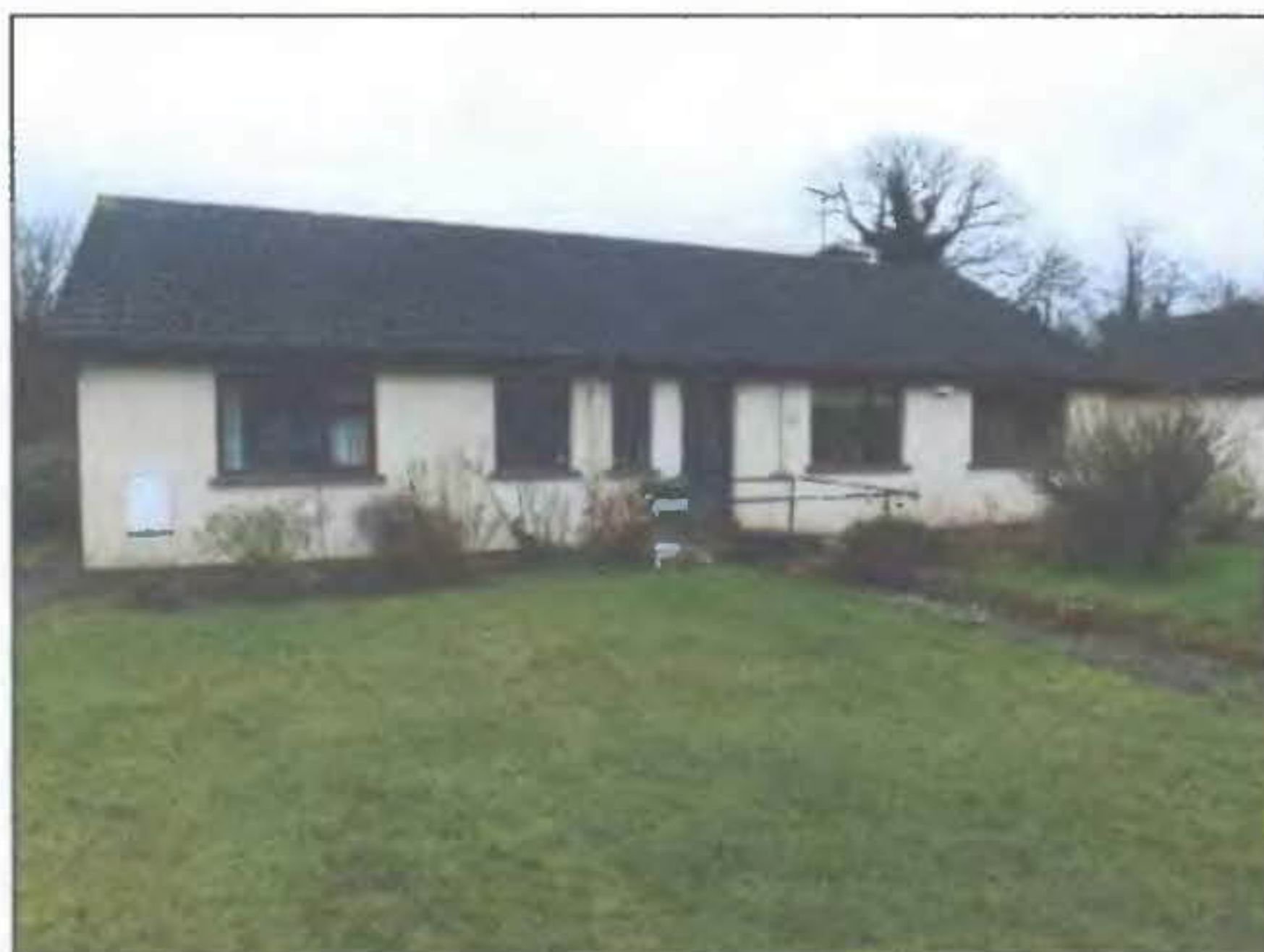
Photo of Rear Elevation
